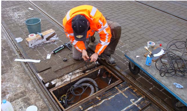
Figure 2 Embedding the sensors into the track
