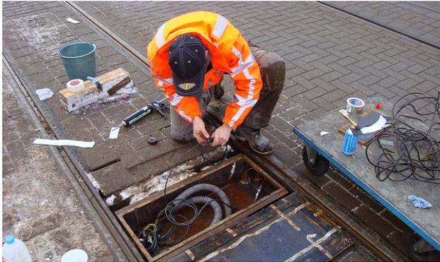
**Figure 2 Embedding the sensors into the track**
